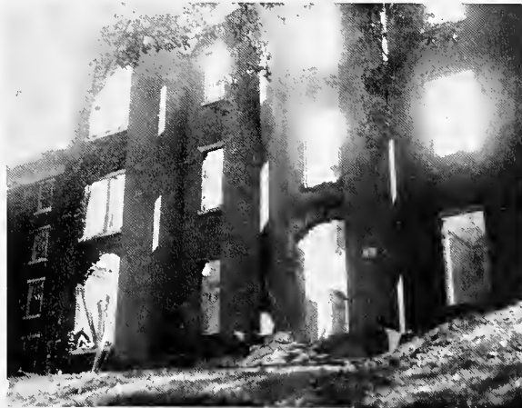
At the Height of the Fire
